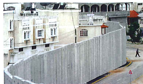
Israeli Security Barrier The Israeli security barrier separates parts of Israel from the West Bank.
