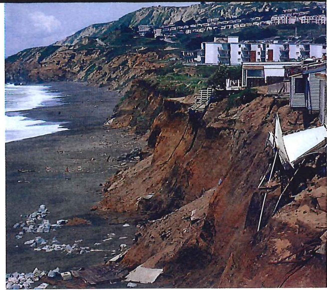
Beach Erosion Ocean waves and tides eroded this section of beach in California.
